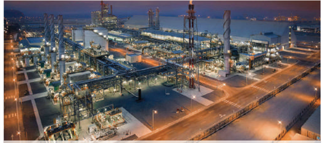
Al Dabbiya Surface Facilities Phase 3 UAE
