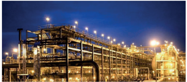
Aramco Jazan Refinery KSA
