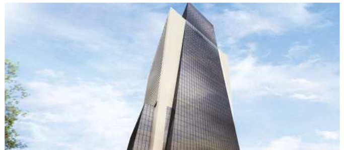
Wafi Hotel Complex and Mall Expansion UAE
