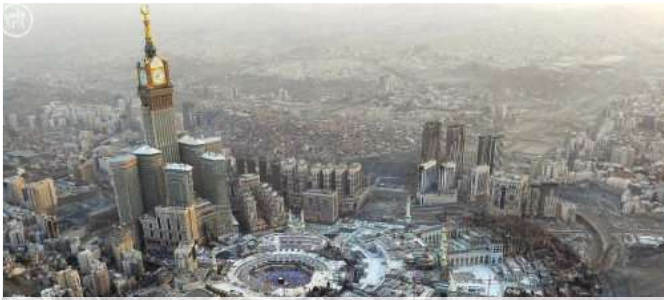
Masjid Al-Haram Expansion Project KSA
