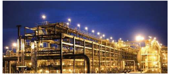
Aramco Jazan Refinery KSA
