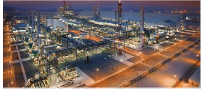
Al Dabbiya Surface Facilities Phase 3 UAE
